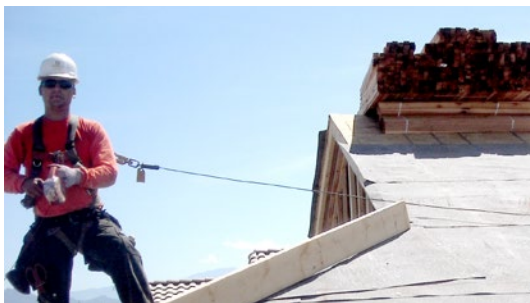
Photo courtesy of ACTA Safety & Peterson Dean Roofing
